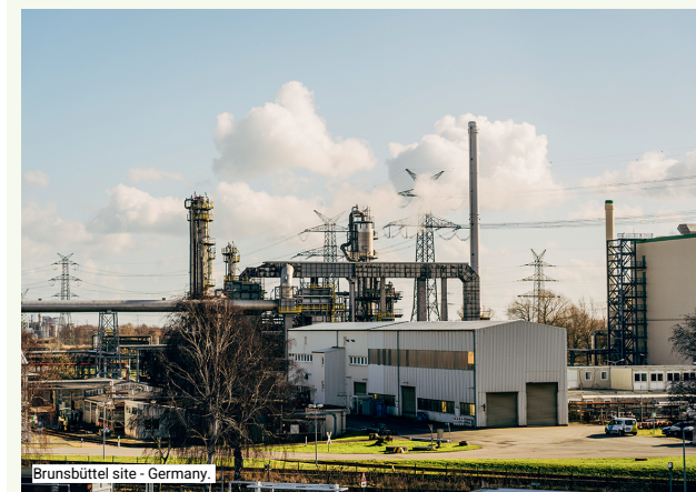
Brunsbüttel site - Germany
