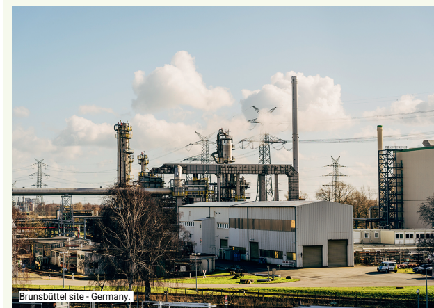
Brunsbüttel site - Germany
